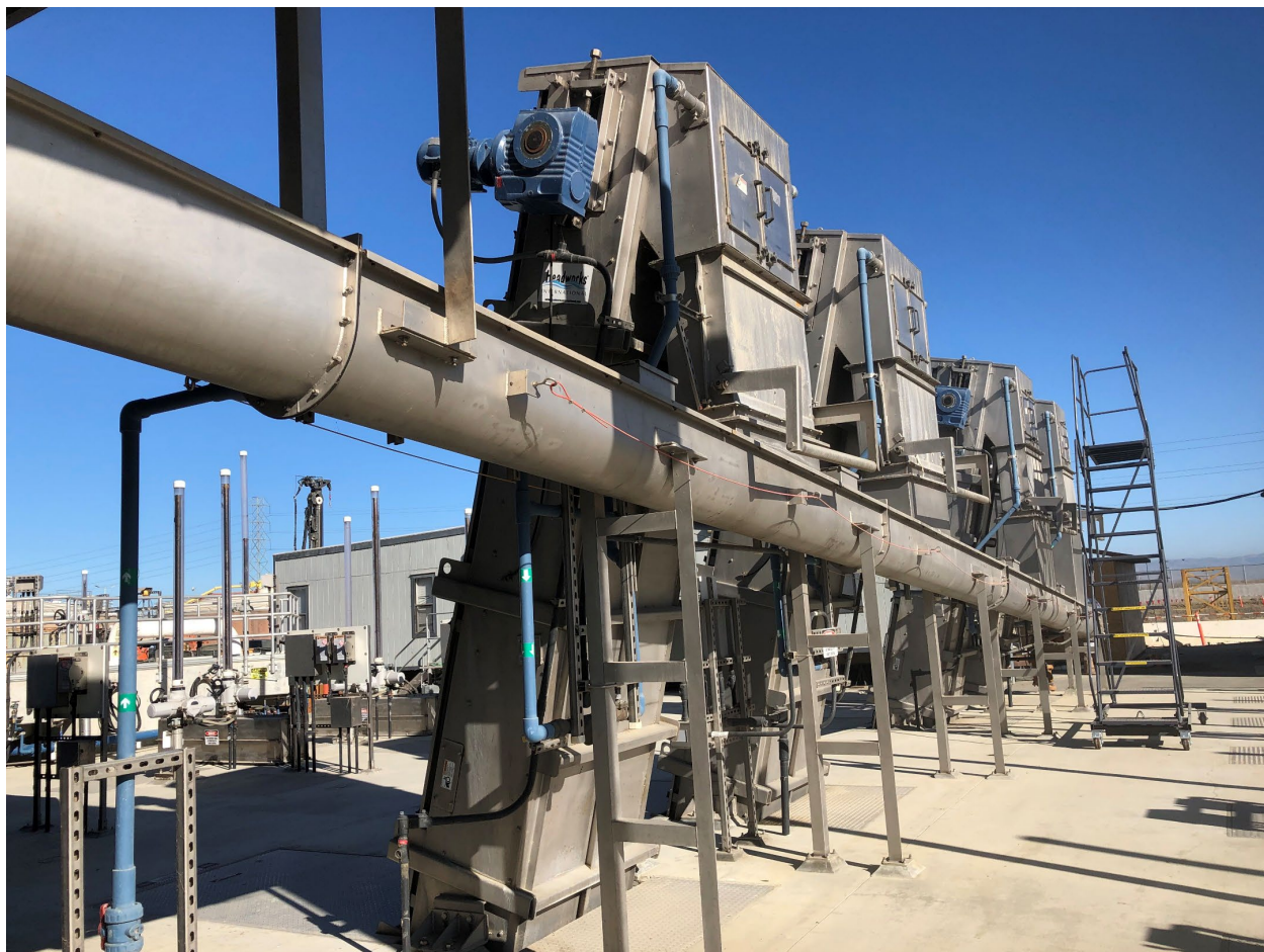
Figure 13.8 Screenings Diverter Gate in Normal Position (Screenings to Washer/Compactor)
