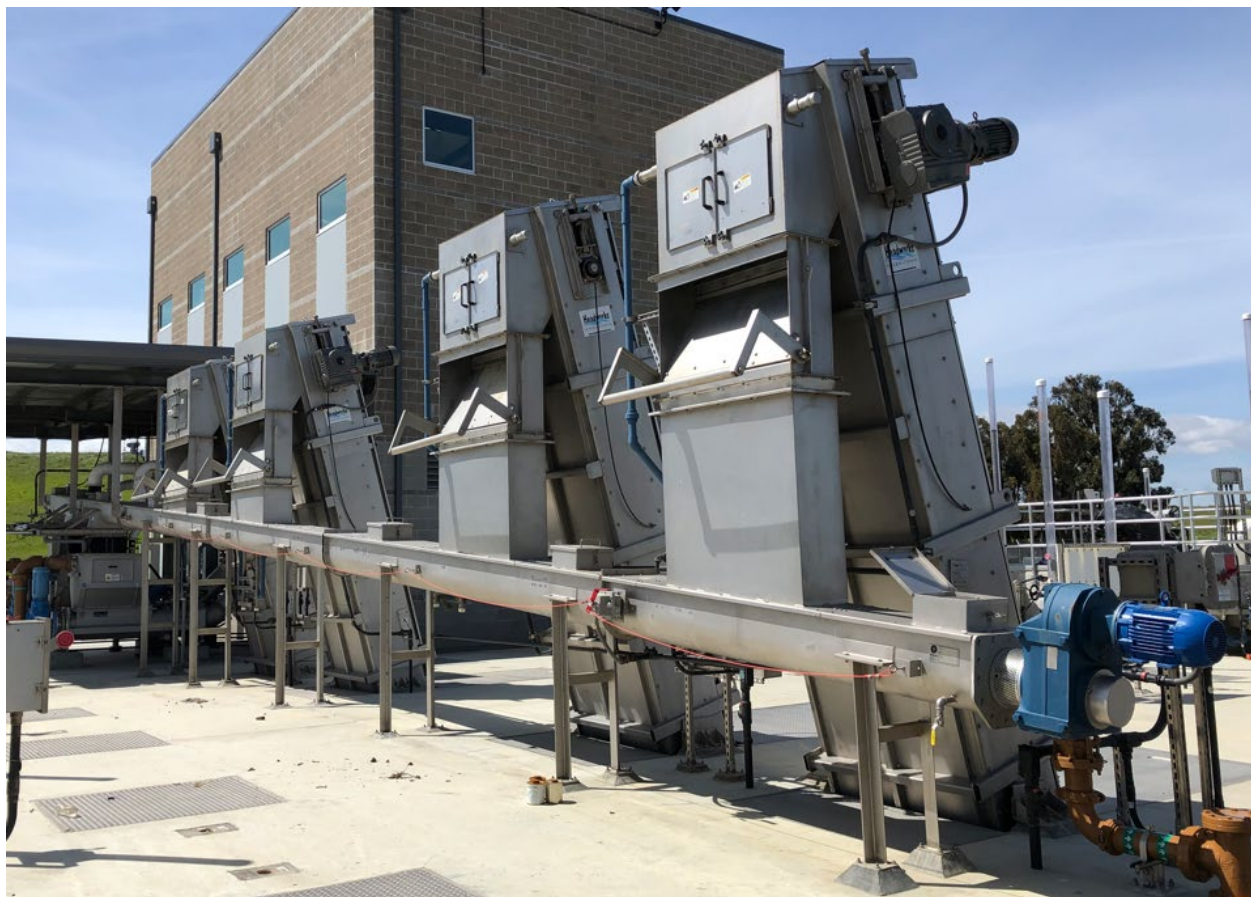
Figure 13.7 Screenings Diverter Gate in Divert Position (Screenings to Dumpster)
