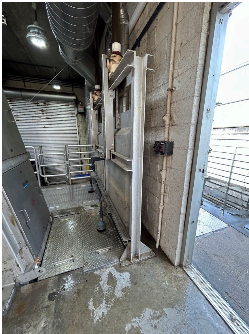
Figure 13.10 Existing Channel Gate
