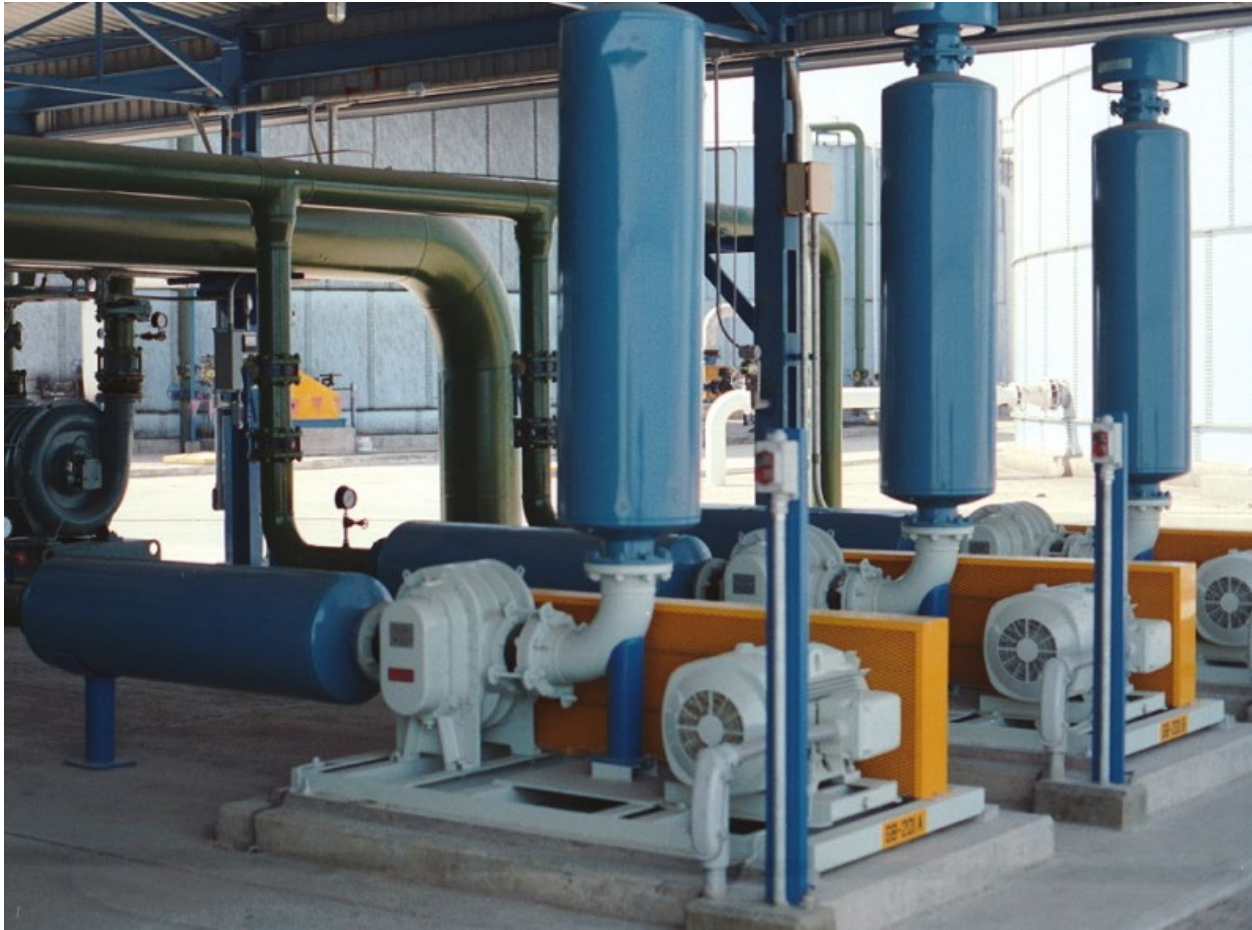
Figure 12.11 Positive Displacement Blowers
