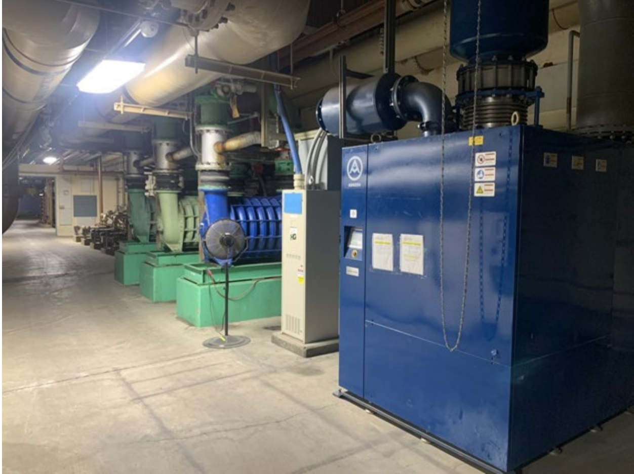
Figure 12.15 High-Speed Turbo Blower at the Durham AWWRF (Right-Most Unit Depicted)
