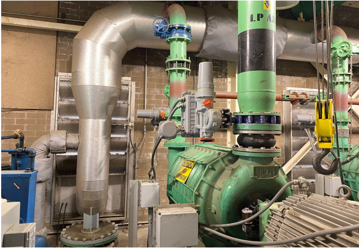
Figure 12.13 Existing Multistage Centrifugal Blowers at the Forest Grove WRRF
