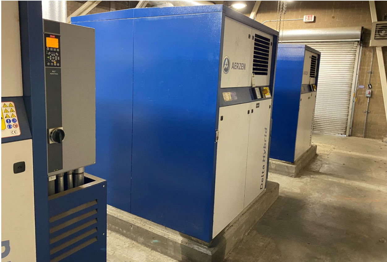
Figure 12.12 Existing Rotary Screw Blowers at the Forest Grove WRRF
