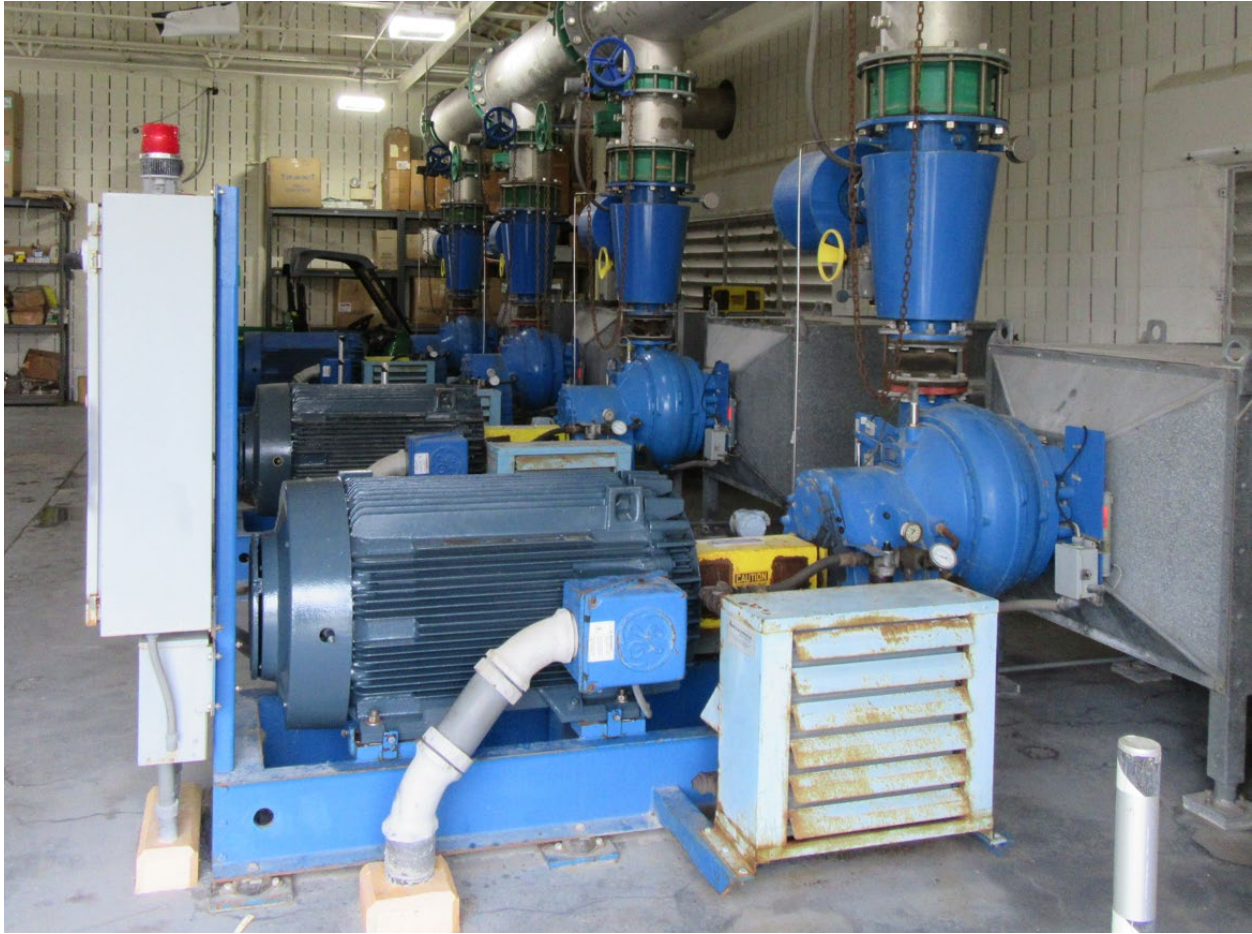
Figure 12.14 Single-Stage Geared Centrifugal Blowers
