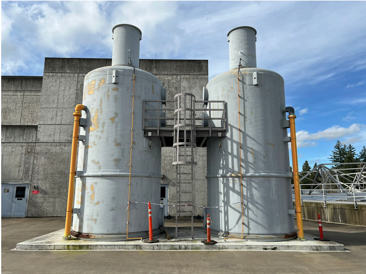
Figure 7.2 Existing Headworks and Primary Clarification Odor Control System
