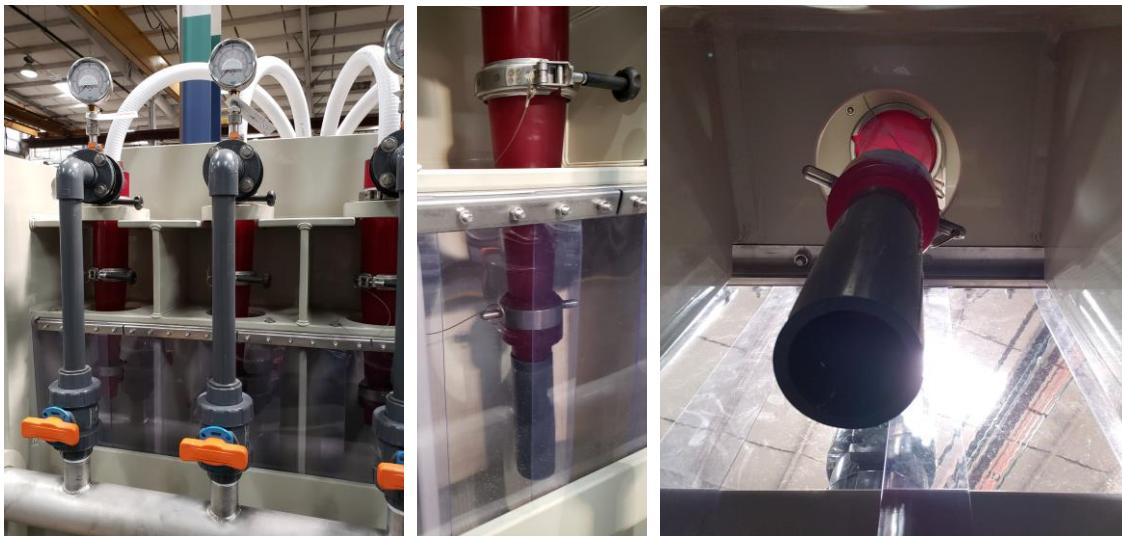
Figure 16 – Installed and Assembled Hydrocyclone / Inside Underflow Box
