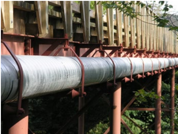
Figure 9.5 Pipeline Attached to a Vehicle or Pedestrian Bridge
