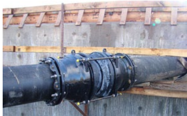
Figure 9.6 Mitigation and Prevention (left = anchoring to prevent lateral shifts; right = flexible joint to allow movement without rupturing pipe)
