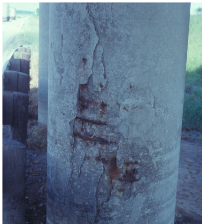
Figure 9.7 Bridge Damage (exposed rebar/spalling)
