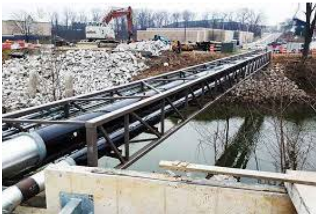
Figure 9.4 Above Ground Pipe Bridge (Bridge Support Pipeline Only)
