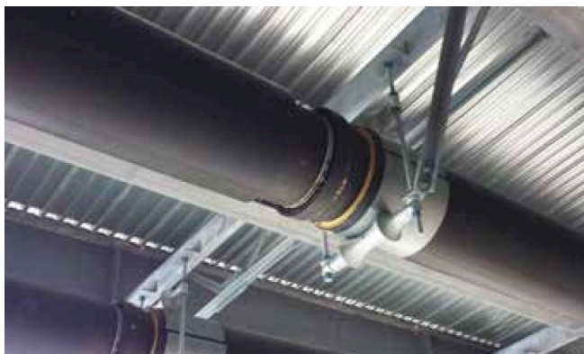
Figure 9.6 Mitigation and Prevention (left = anchoring to prevent lateral shifts; right = flexible joint to allow movement without rupturing pipe)
