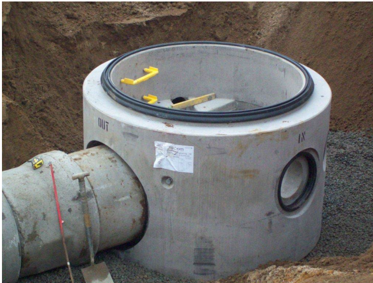
Figure 9.8 Flexible Pipe Connection Manhole
