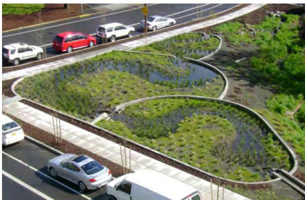
*Headwaters at Tryon Creek, SW Portland. The rounded and stepped design of these infiltration planters are molded to the specific conditions of the site. The concrete walls are a creative interpretation of check dams that are used to convey water across flat surfaces over steep topography.*
