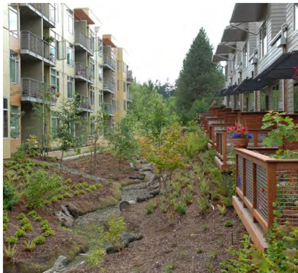
*Headwaters at Tryon Creek, SW Portland. Headwaters is a residential development where senior housing, town homes, and an apartment building were designed to be integrated with the daylighting (removal from an underground piping system) of a tributary of Tryon Creek.*
